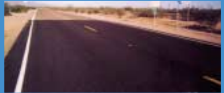
Rt 238, Maricopa County, black area shows TOR plus GTR dry process
