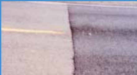
Maricopa County, Arizona. Left side, chip seal. Right side, TOR plus GTR.
