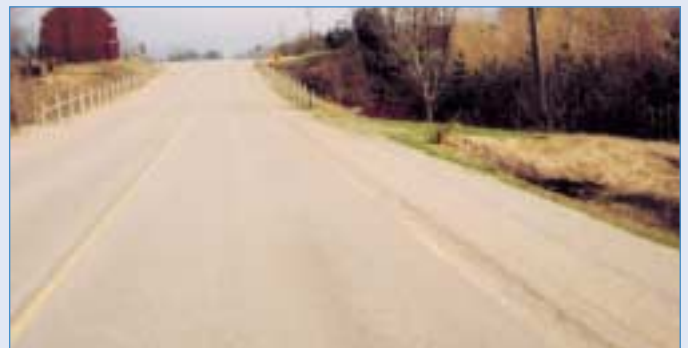
Rt. 7 Owen Sound, Ontario, paved with TOR plus GTR, no cracks after 4 1/2 years.
