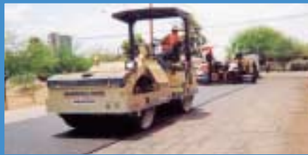
Phoenix, Arizona. On left paving with TOR plus GTR.
