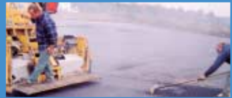
Lincoln, Nebraska parking lot paved with 100% RAP.
